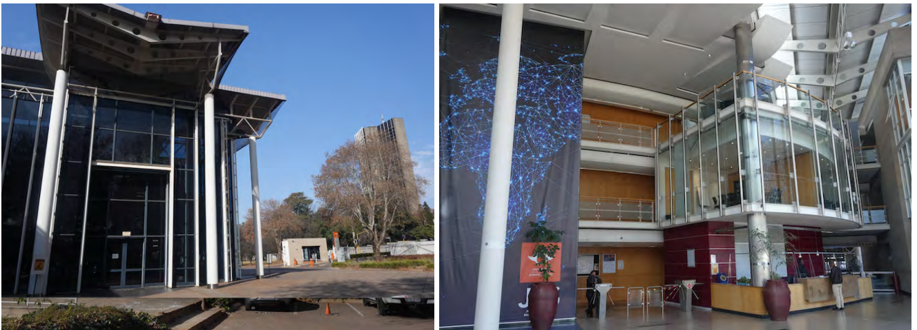
Johannesburg Business School entrance gate and lobby.
